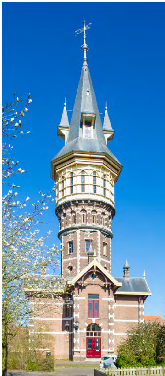
Schoonhoven, Watertoren (foto Arjan Bronkhorst)
